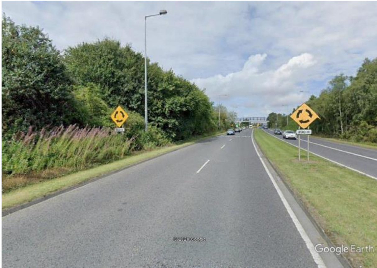
Figure 6-53 – Existing Road Layout on Finglas Road northbound between Mellows Road and St. Margaret’s Road
