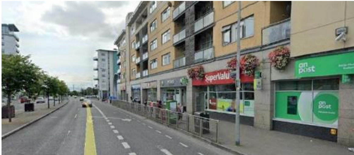
Figure 6-4 – Ballymun Main Street West
